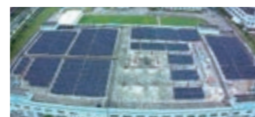
Solar panels at OHARA OPTICAL (ZHONGSHAN) LTD.
